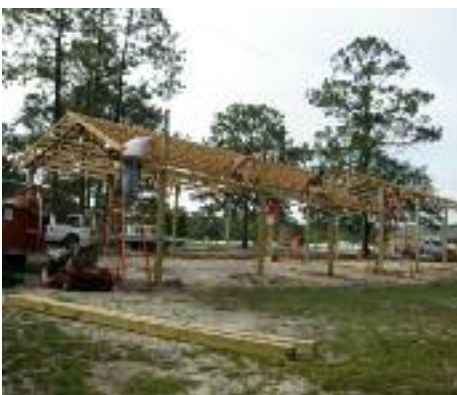
Watching the Roofers
