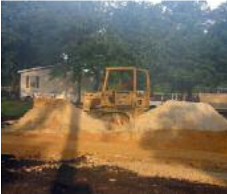
Grading the Land
